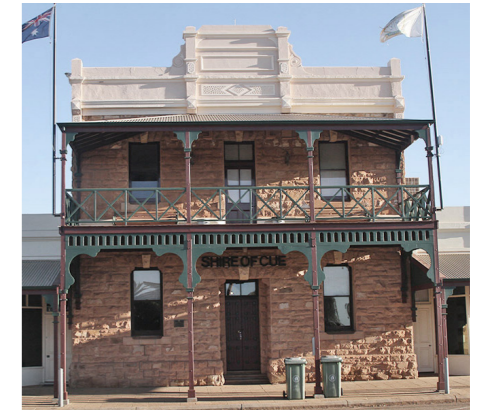
Cue Shire Offices
